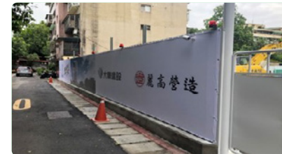
Perimeters of the construction site are fenced off and pedestrian safety corridors are established to prevent soil dust pollution and ensure pedestrian safety.
