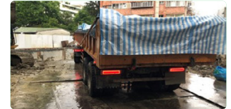
Sealed trucks are used to transport wet soil or when transporting dry soil, the vehicle is covered with dust-proof plastic sheets to prevent soil dust pollution during the transportation of waste soil.
