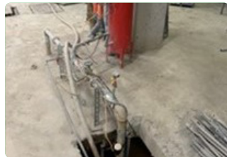
Collecting surface runoff water on the 1 st floor and re-directing it to the raft foundation for use as construction site water source.
