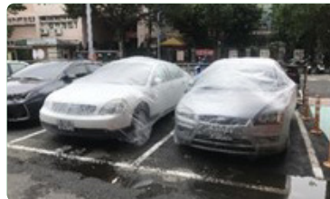
During the pouring of structural floors, protect the surrounding roads and parked vehicles on the construction site to minimize pollution to nearby vehicles.
