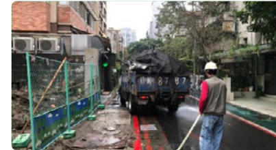
A car wash station and high pressure washing equipment are set up to prevent vehicles from carrying dirt or other pollutants when transporting waste materials, thus avoiding soil and air pollution in nearby communities.
