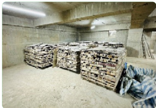
Formwork material classification, promoting reuse and reducing disposal.
